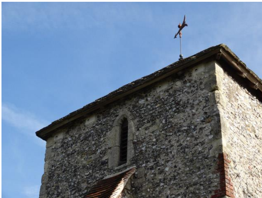
St. Botolphs: Swift nest chambers installed below the eaves
